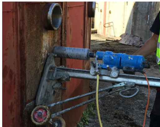
Fig. 2. View of specimen coring from concrete containment wall.
