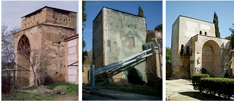
Figure 1: The Gate of Burgos, from left to right: South façade: in 2003; after the 2005's collapse; in 2012, after its restoration.
