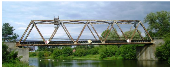
FIGURE 1. Railway truss bridge in Nieporet near Warsaw
