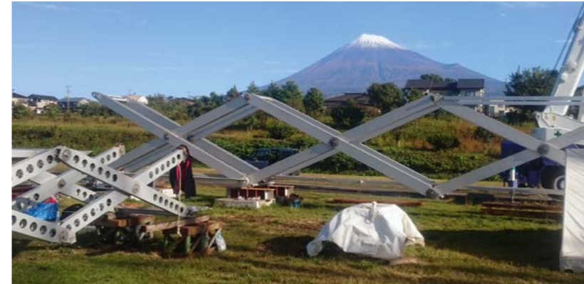
Fig. 10.11. View of the scissor-type bridge prepared to perform dynamic research carried out in cooperation with IPPT, Fuji, JAPAN
